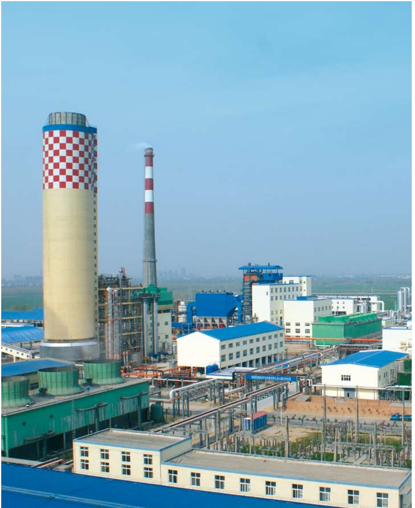
Third plant near completion with 400k tons urea and 50k tons methanol annual production capacity
